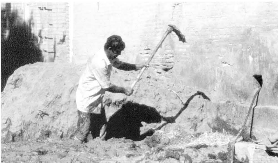
Preparation of the wall finishing, i.e., mortar of mud and straw
