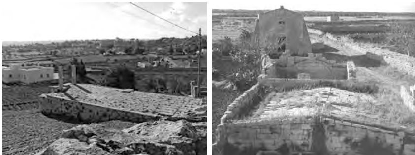
Fig. 6-8. Model and images of rural semi - hypogean cisterns with trough typical of the "murgian" country. (author: C. Montalbano)
